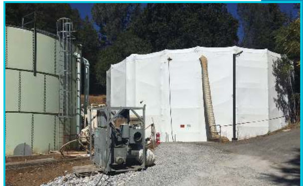
Columbia Clearwell Project
