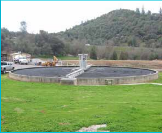
Center cans installed at the Regional Facility
