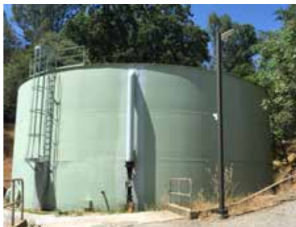
Current Columbia Clearwell Tank
