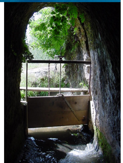
The O'Neil Tunnel Improvements Project
