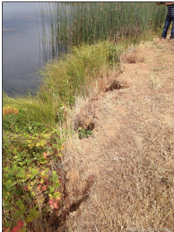
Erosion on the Earthen Dam
