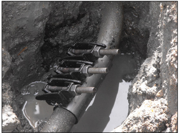
Construction/Maintenance Crews Repairing a Leak on Willow Springs Drive
