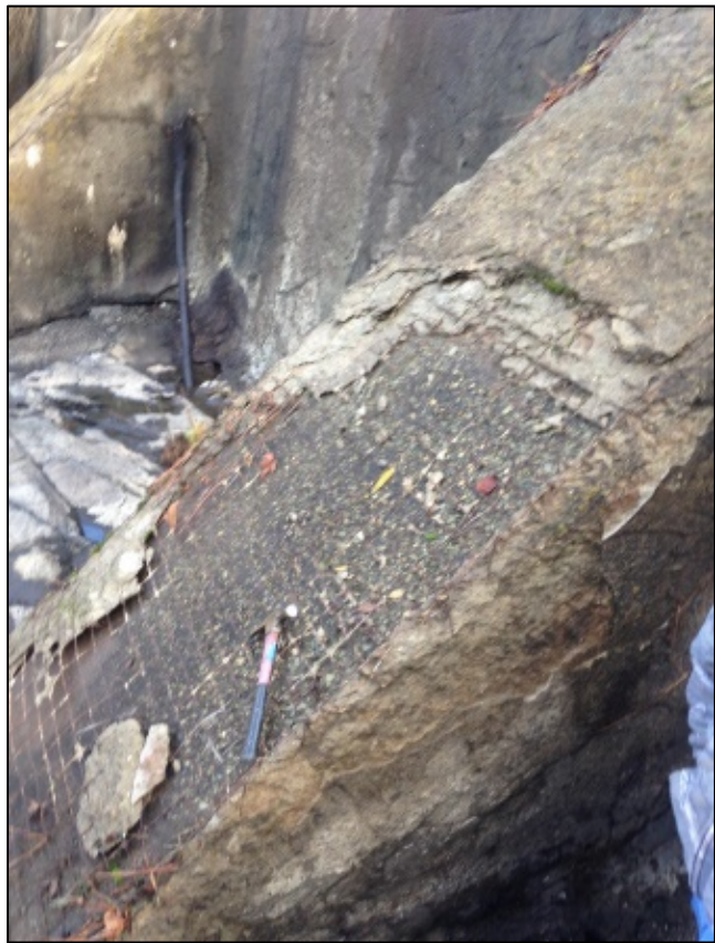
Concrete Spalling on Spillway
