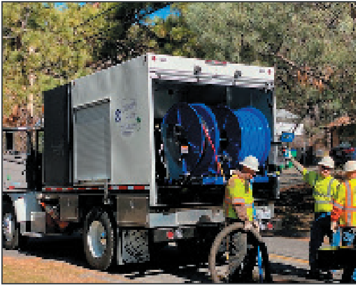
Flushing sewer pipelines before assessment
