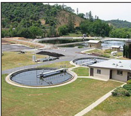
Sonora Regional Wastewater Treatment Plant
