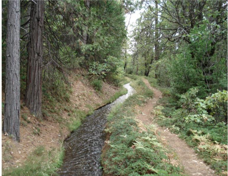
A key component of the Tuolumne Utilities District's (TUD) water supply infrastructure is the ditch system. The original ditch system was conceived and constructed by a group of energetic and resourceful miners in the early 1850's to deliver water to the communities and miners in Sonora, Jamestown, and Columbia.
